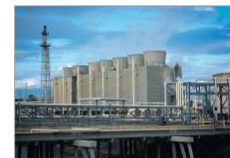
Oxidizing Microbiocide For Cooling Water Systems
