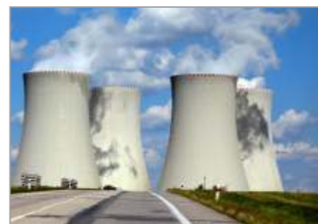
Power Plant - Cooling Towers
